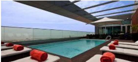
Swimming Pool and WWTP in Baía Hotel, with water recovery for irrigation Client: Teixeira Duarte Angola
